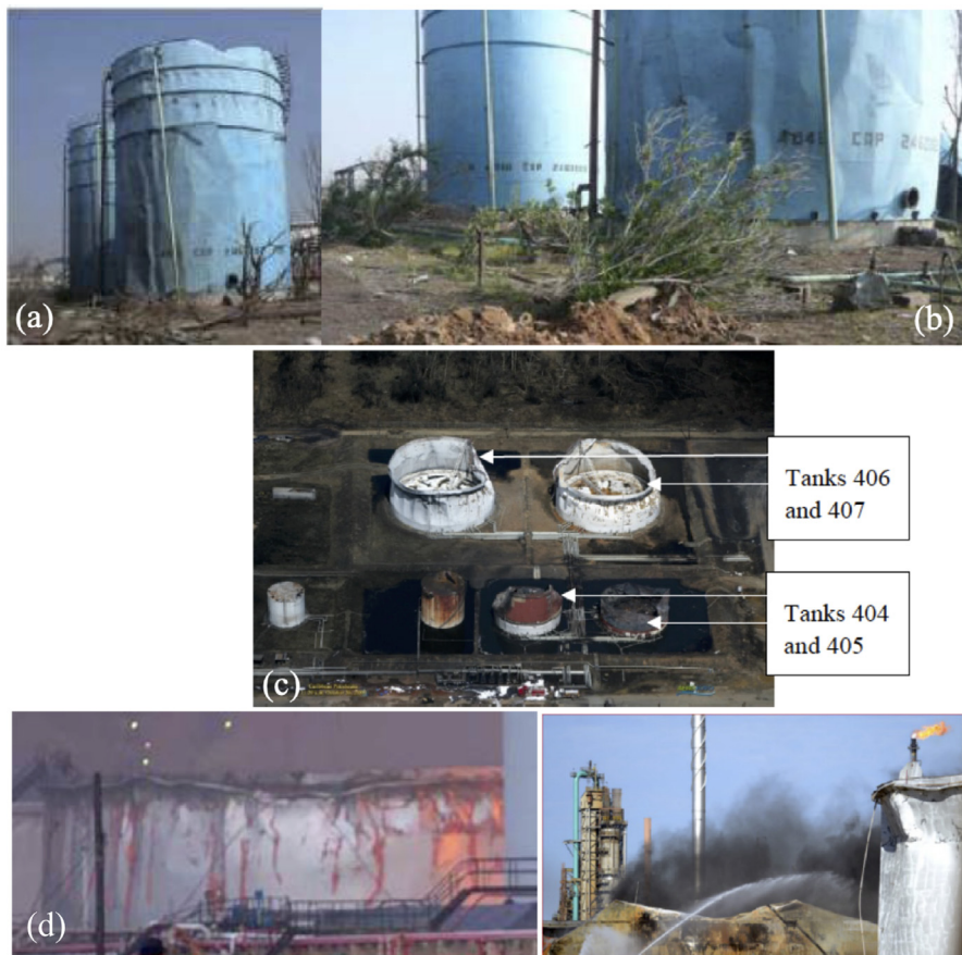
Fig. 21. Views of a crushed, empty firewater tank at Jaipur (a) from a distance and (b) close by Johnson [6]. Empty tanks at (c) Puerto Rico [5] (reproduced by permission of the Fire and Blast Information Group, (FABIG), www.fabig.com ) and (d) Amuay [50].
