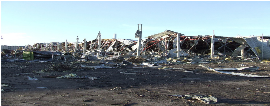
Fig. 25. The destroyed south side of the Fuji Building at Buncefield. The building was on the west side of an open car park [3].
