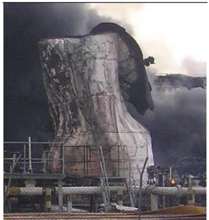
Fig. 20. Crushing damage to partially empty tank 601 at Buncefield [49].
